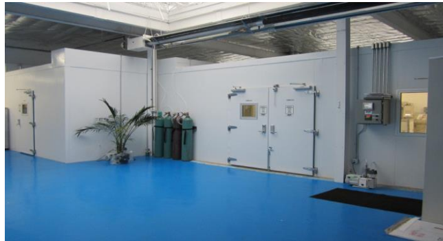
One of the 4 battery-grade dry rooms at HBC/G 3
